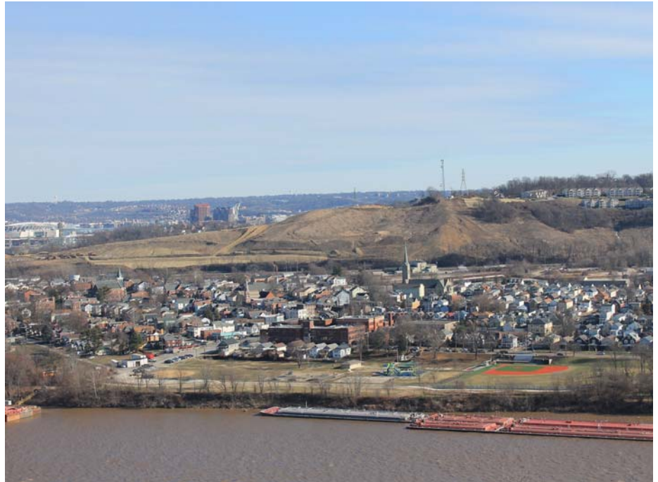
Ludlow, KY hillside post-cutting - January, 2024
