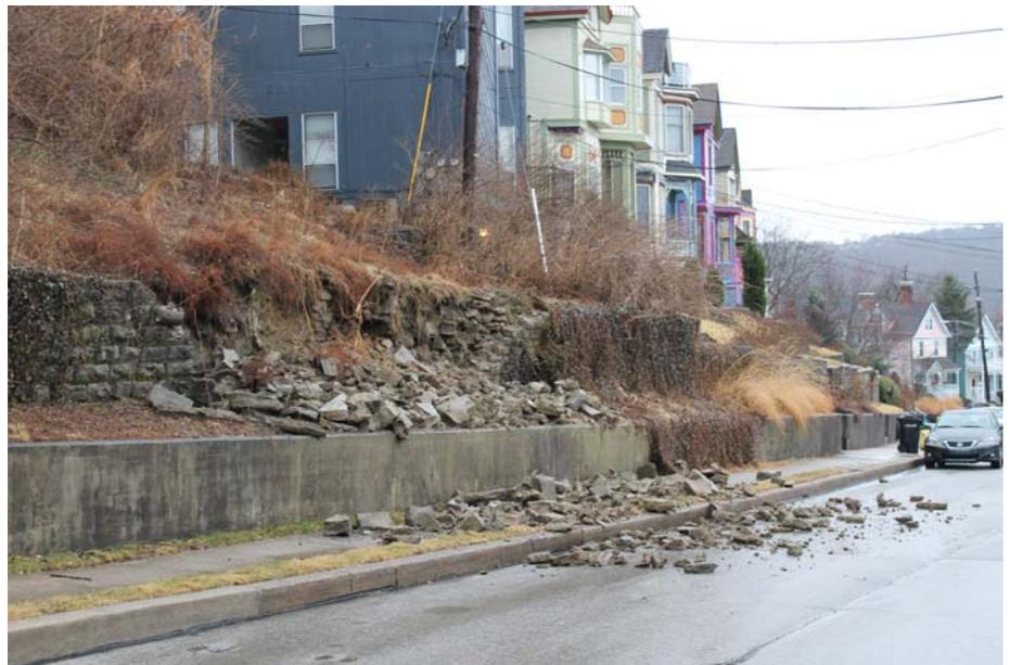
***Slope failure damages a retaining wall in Mt. Lookout***
