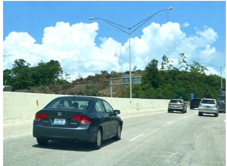
Silverton hillside in process of being flattened
